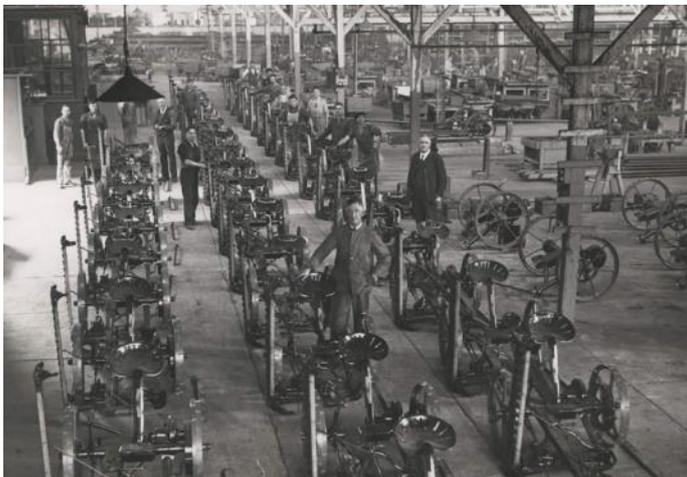
*A mower assembly line on the factory floor of Melbourne's Sunshine Harvester factory, which made agricultural machinery.
